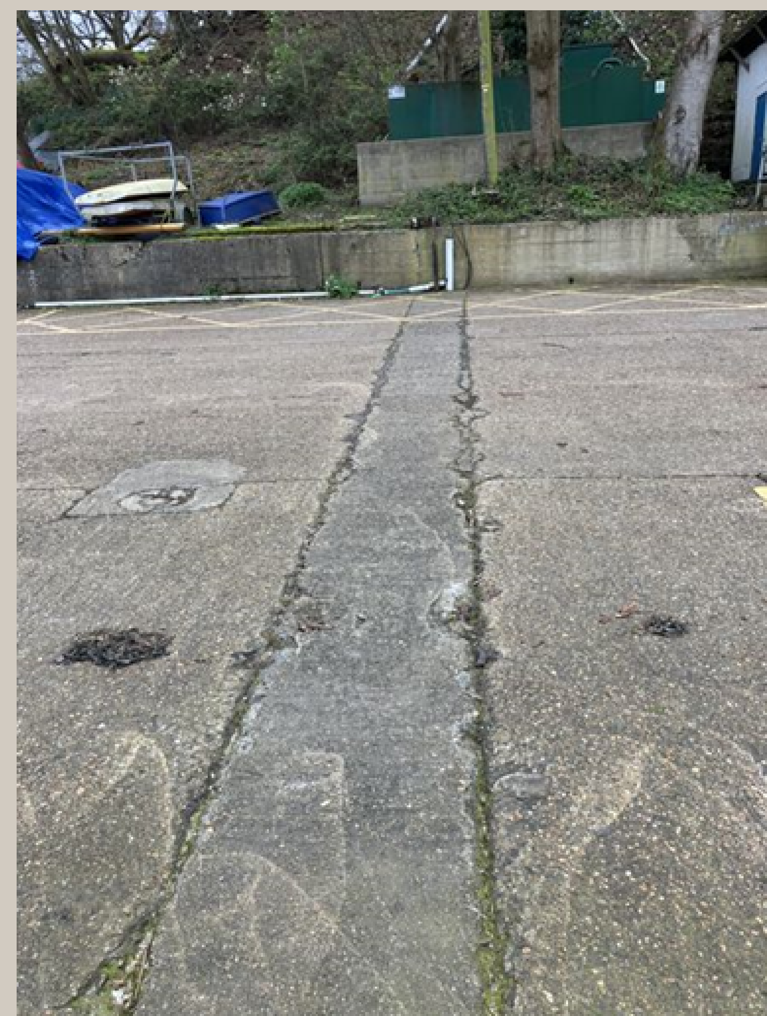
7. Channel, now concreted over, for diesel pipe to dolphins.
