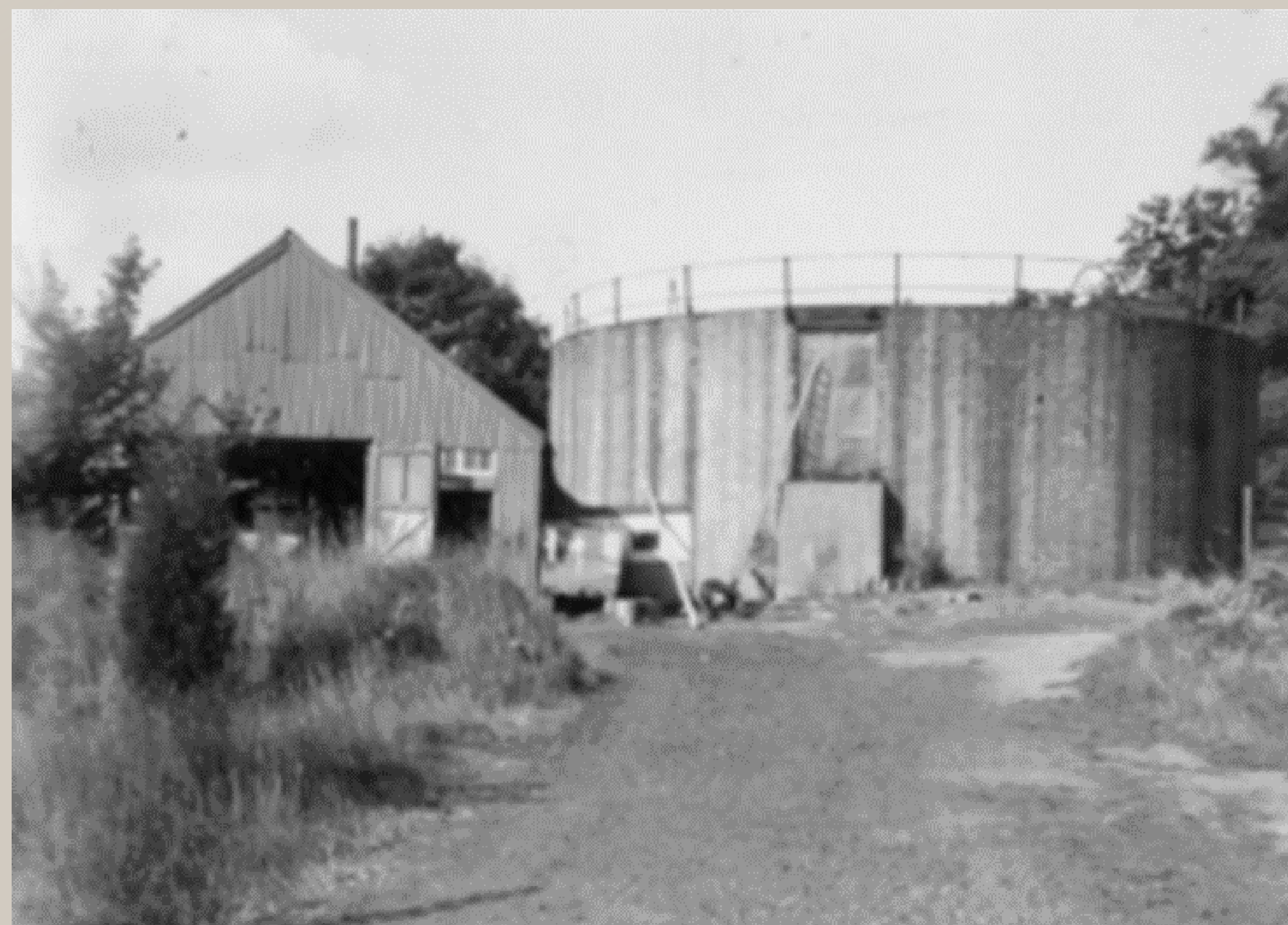
Lower diesel storage tank c. 1950
