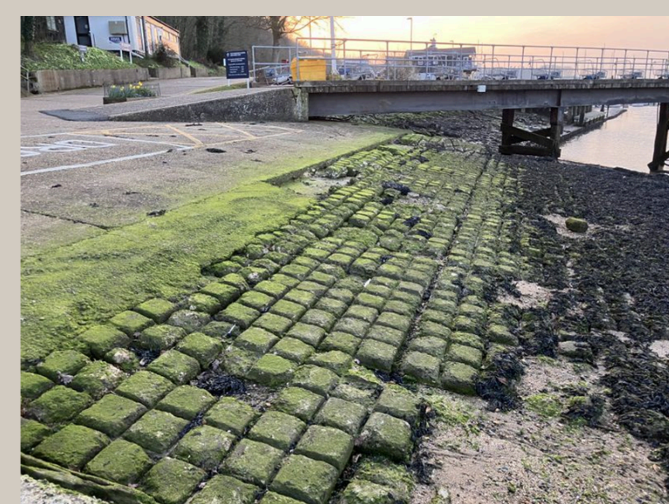
11. Flexible matting – chocolate blocks - in the intertidal zone. Much of the matting has disappeared as it no longer reaches to low tide. The matting was mostly laid in 15 block sections, 3 x 5. 62 cm (24 in) x 102 cm (40in). The mats are 12.7 cm (5 in) thick. Each block is of a similar design of moulded concrete.
