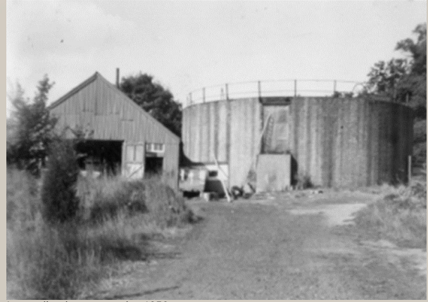
Lower diesel storage tank c. 1950
