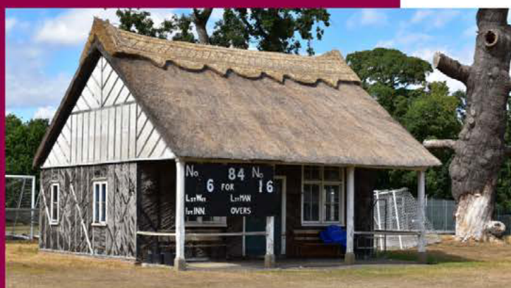
PRESENT: THE NEW THATCH WAS COMPLETED IN SUMMER 2022
